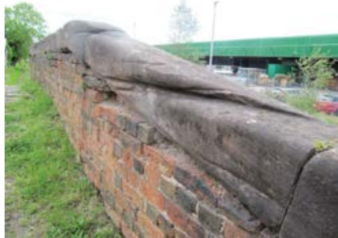
The canal arm bridge with rope marks
