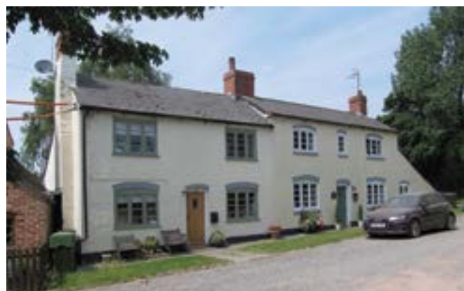
The Machine House to the right
