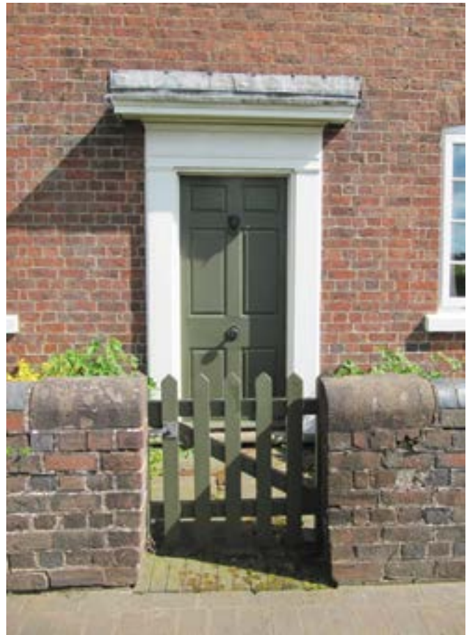
Canal cottage gate and doorway
