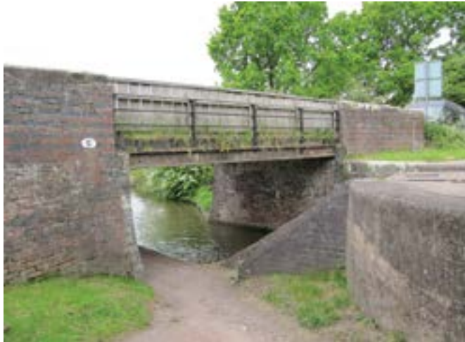
Bridge at Upper Gambolds
