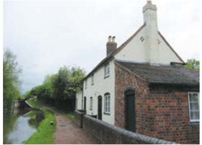
Lock keepers cottage, Stoke Pound
