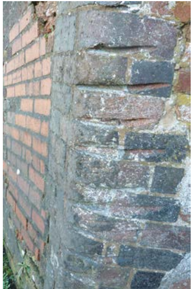
Rope marks on a bridge wall
