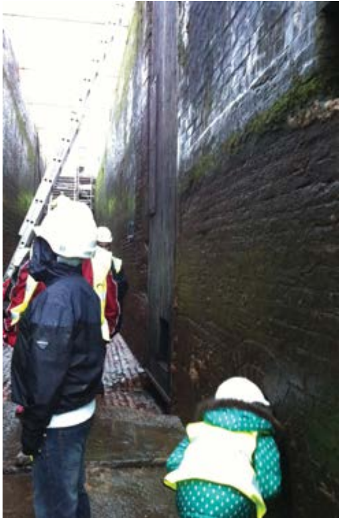
Lock 58, emptied for repairs
