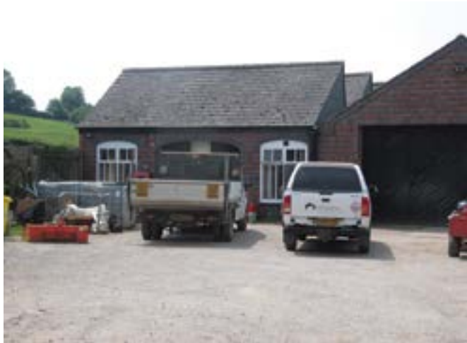
SND building at Tardebigge Basin
