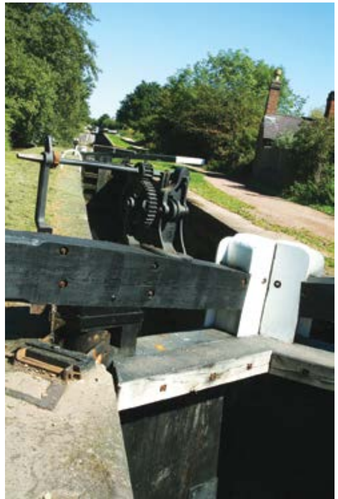
A section of Tardebigge Flight looking in a north easterly direction with Reservoir Cottage on the right
