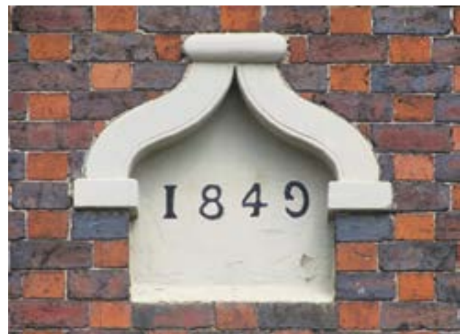
Navigation Row construction date
