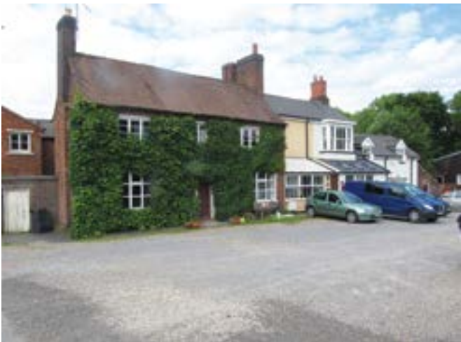
Wharf Cottage adjacent to Bottom Lock, originally Weighbridge House and toll office
