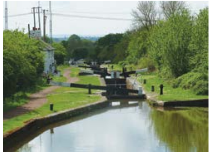
View from Lock 51, looking south west
